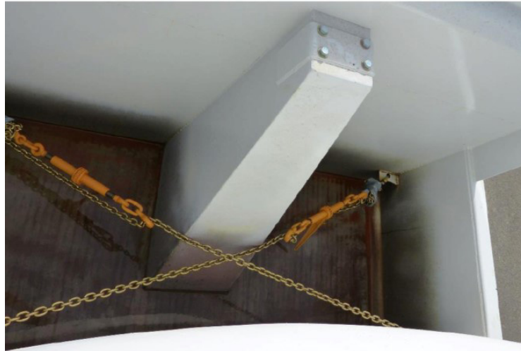
Figure 14 – Front Chains Option (viewed from above)
